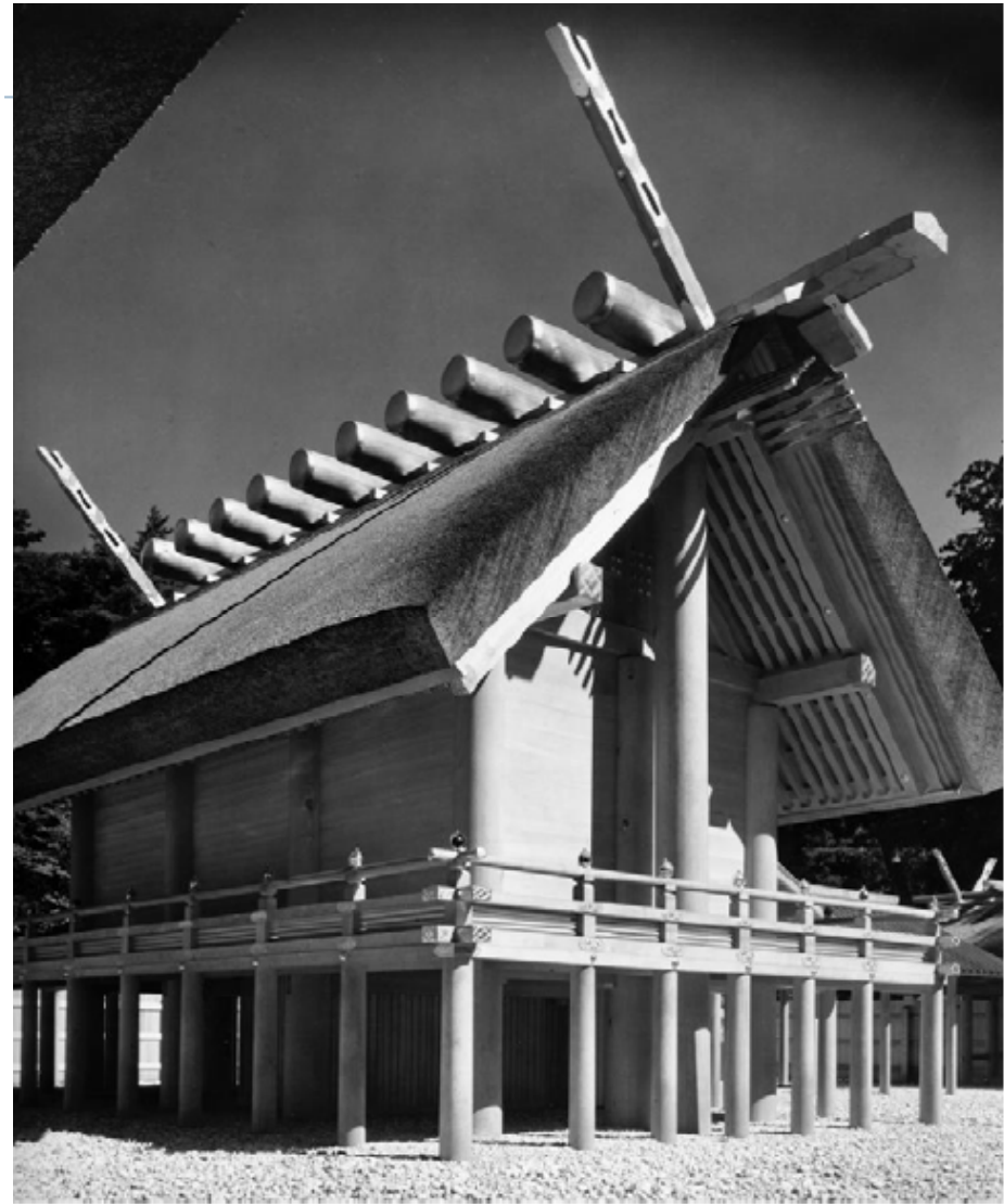
Fig.1 Main Building of ISE Shrines photo:Y. Watanabe
